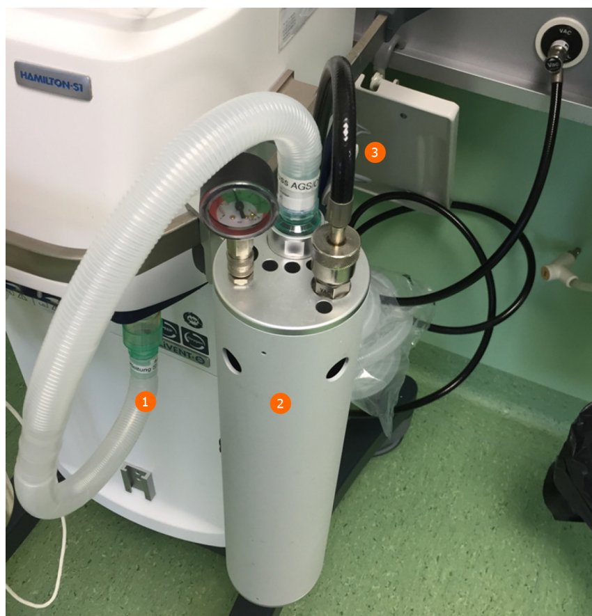
Figure 6 Example of a vacuum-based gas scavenging system (CleanAir™ system). 1 Expiration port of the ventilator; 2 Open reservoir scavenging system; 3 Vacuum line.
